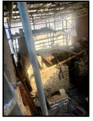
The old Ferryman's Cottage on Beach Road is undergoing change! In the photo you can still see the chimney on the left and a blocked up window at the back has been made into a doorway. The roof has been removed and will be replaced using as many of the old small slates as possible. Hard to say what was holding the roof up really, all the roof rafters were rotten. The front of the
